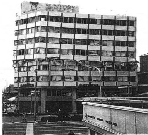
figure 1: progressive collapse of middle class of building as a result of Kobe Earthquake, 1995
