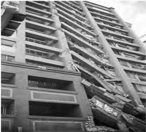
figure 2: progressive collapse as a result of Taiwan Earthquake, 1999
